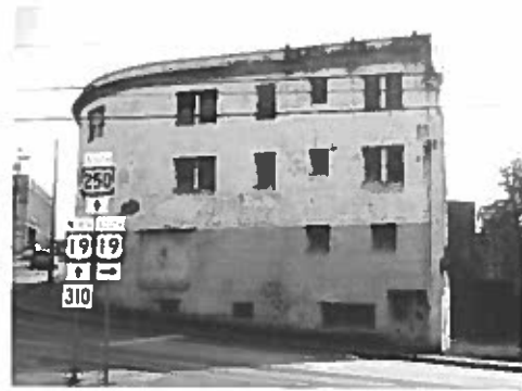
Photo 1: Fairmont Tire Center – Vacant building in downtown Fairmont
