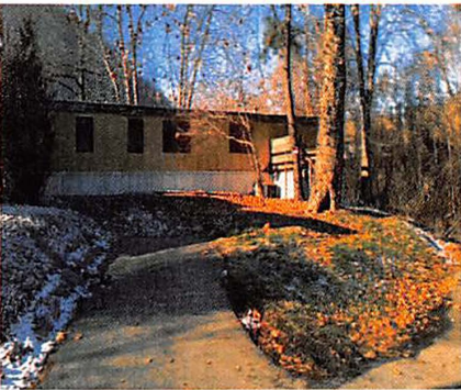
Howard Avenue- Privately Owned, Vacant and Dilapidated
