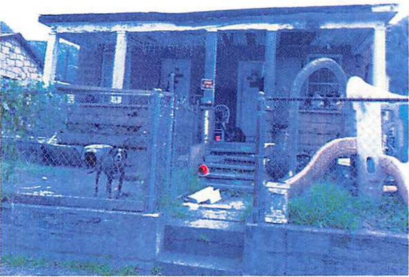
Parcel 37: 143 Orchard Avenue, Owner Occupied, Dilapidated, Chronic Ordinance Violations
